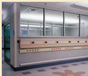
WASHINGTON HOSPITAL CENTER NEONATAL INTENSIVE CARE UNIT
